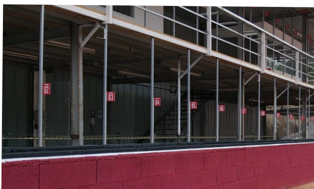
Driving Stand Stairs
